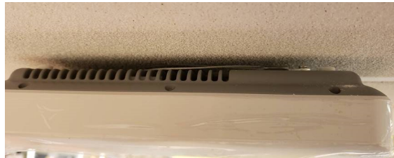
FIGURE 6 Tucking Excess Cable
