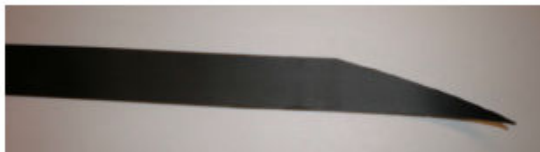
FIGURE 16 Cutting the Sealing Tape at an Angle
