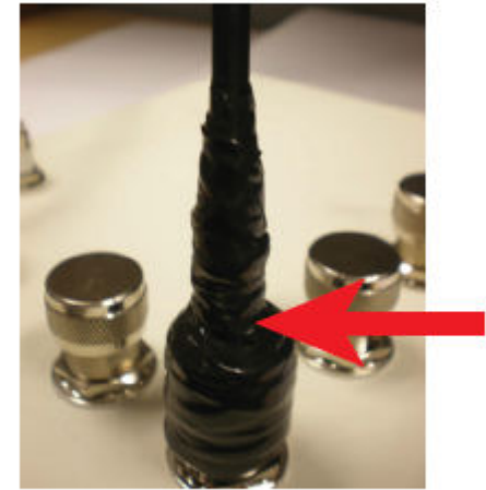
FIGURE 19 Wrapping the Electrical Tape
