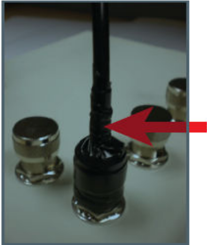
FIGURE 15 Wrapping the Electrical Tape
