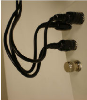
FIGURE 21 Creating Cable Drip Loops
