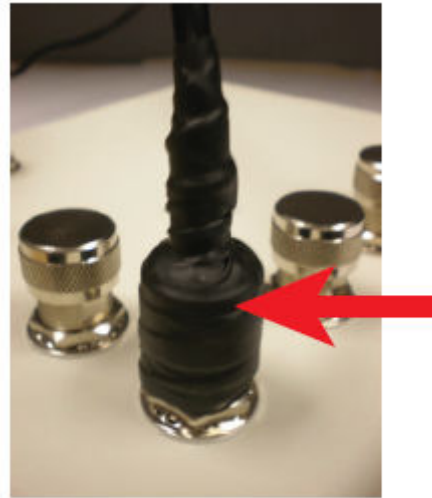
FIGURE 17 Wrapping the Sealing Tape
