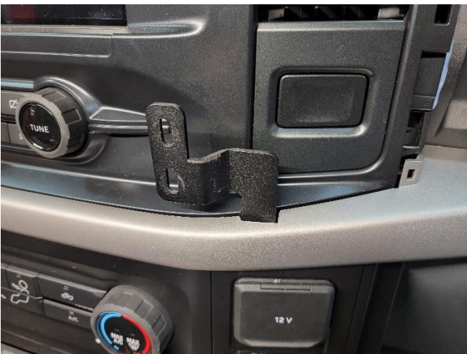
Reinstall previously removed trim.
