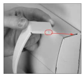
Step 2. Snap DS4000C Cover sections onto DS4000B Raceway Base and align with DS4010B Blank End Fitting.
