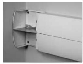
Step 4. Snap DS4010A Cover straight on. Cover will overlap DS4000C Raceway Cover
