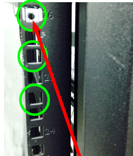
Insert nut in each front post
