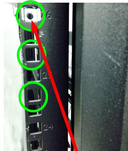
Insert nut in each front post
