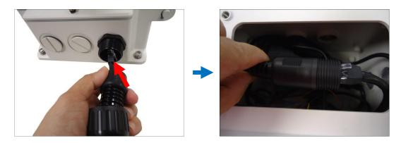
3. Secure the flex conduit fitting onto the junction box hole.
