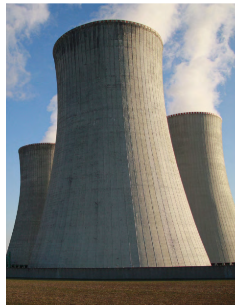
Figure 1. Cooling towers at a nuclear power plant
