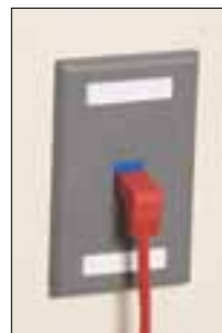
Down cable: Cable clip faces down and the cable angles down. Shown: EVNSL23E-0003-DS EVNSL23E-0003-DS
