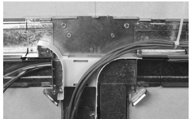
COVER INSTALLATION: Hook corners as shown and snap into place.
