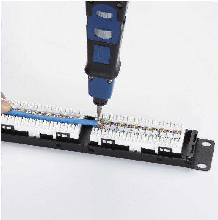
Figure 2. Terminating the wire conductors.
