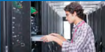
Backup Power UPS
