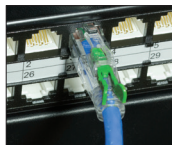
Figure 3. Squeeze the butterfly tabs and pull back to release the pin.
