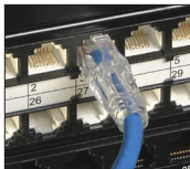
Figure 1. 3-Series Patch Cable (empty—no pin) in RJ-45 port.
