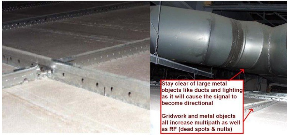
Figure 26: Installing AP above ceiling tiles: Pick an area clear of obstructions, avoid ceiling clutter
