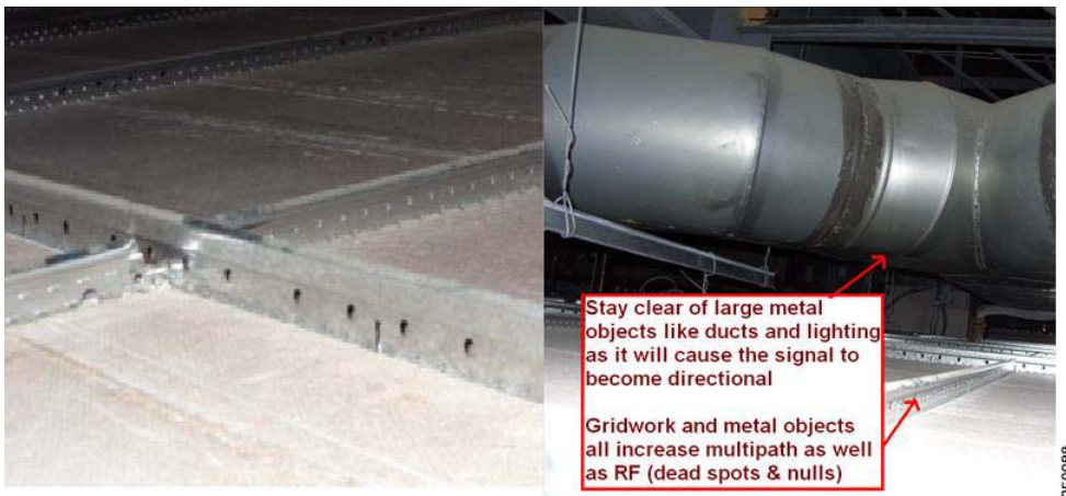
Figure 22 Installing AP Above Ceiling Tiles: Pick An Area Clear of Obstructions and Avoid Ceiling Clutter
