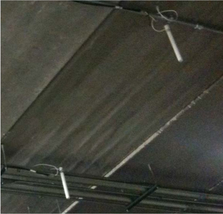
Figure 51 Antenna Placement- Avoid Spacing Antennas Further than 10 Ft (Antennas Should be in the Same RF Coverage Area)
