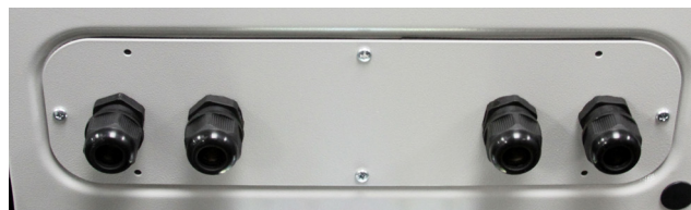
Battery Platform on Floor of Enclosure
