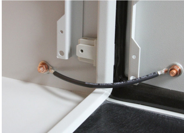
Grounding Cable Installed
