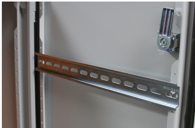
DIN Rail installed on door
