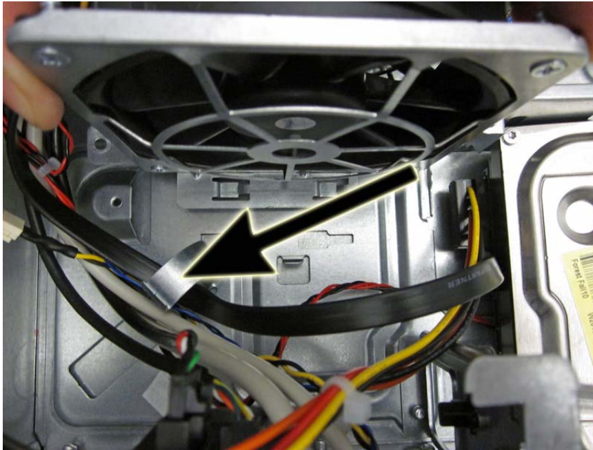
Figure 8-28 Removing the cables from the clip
