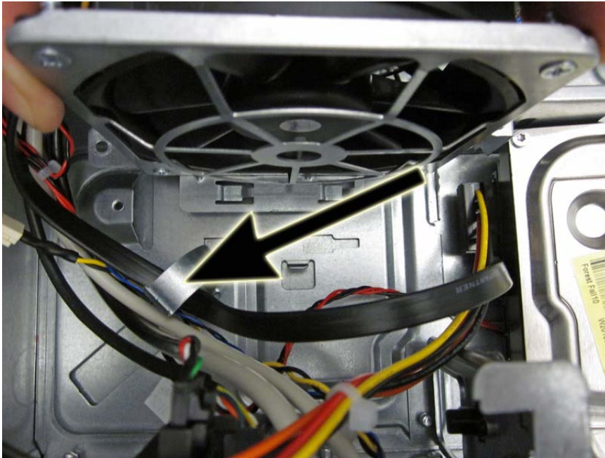
Figure 8-27 Removing the cables from the clip
