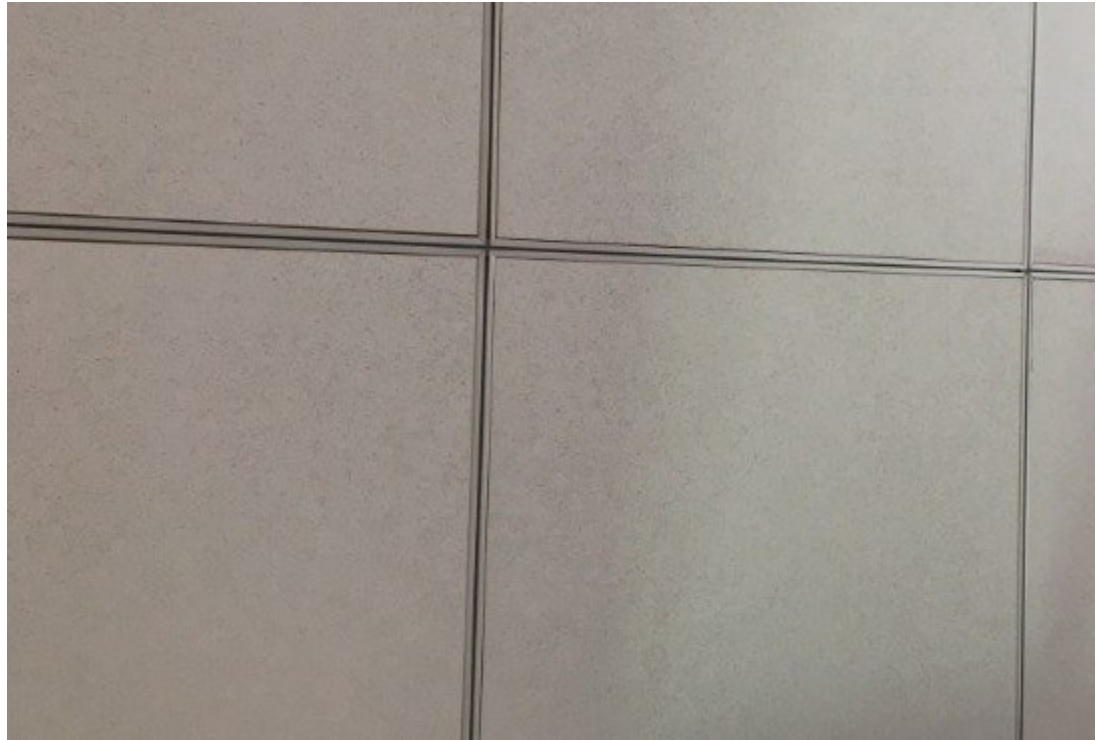
Figure 14: Example of Channel Rails used on thin rail (recessed rail) ceilings
