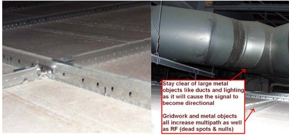
Figure 26: Installing AP above ceiling tiles: Pick an area clear of obstructions, avoid ceiling clutter
