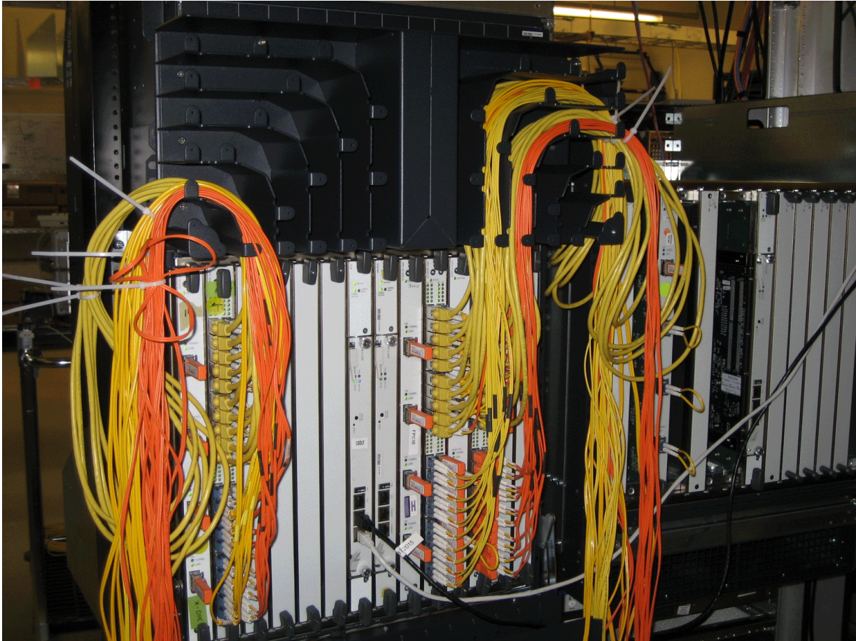
Figure 109: Dressing the Cables Through the Routing Channels
