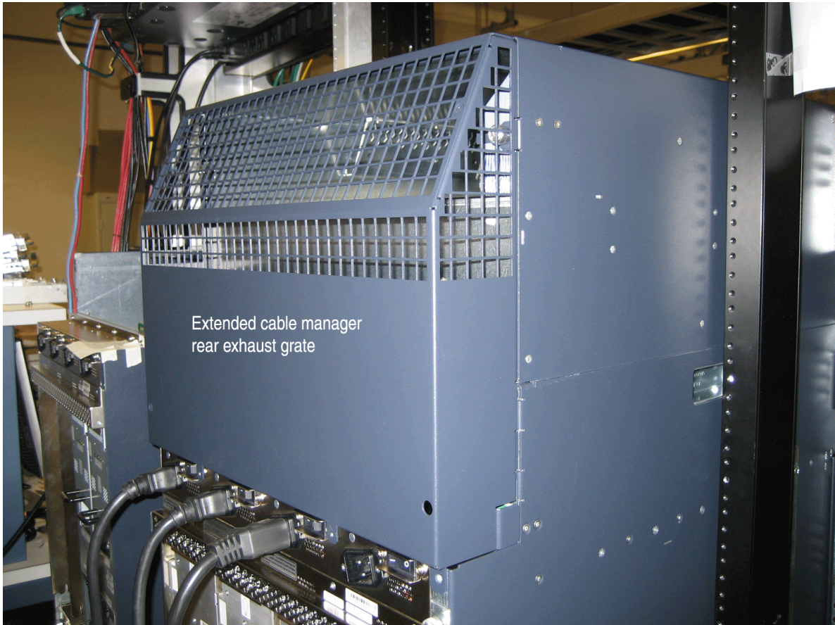
Figure 102: Installing the New Rear Air Exhaust Grate
